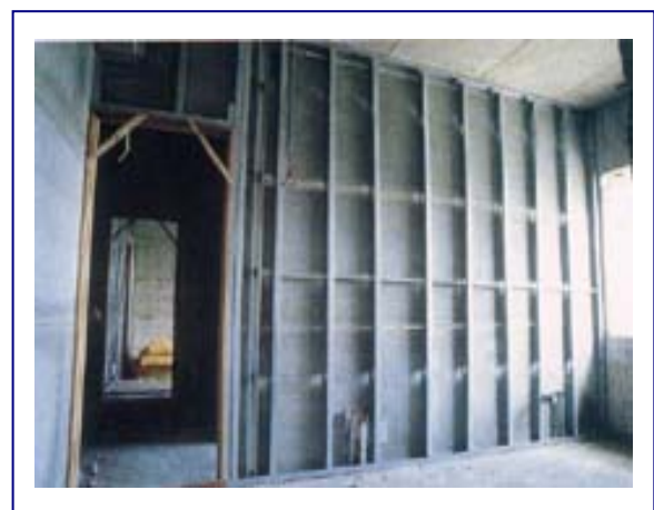
▲ 輕鋼架隔間牆施工中案例
